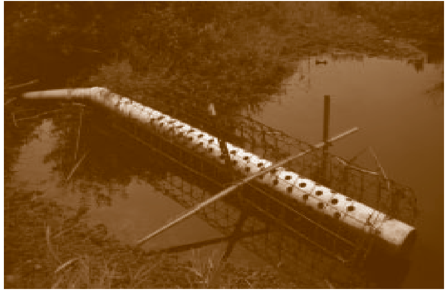
Figure 2. Water level control device. These devices are likely to fail if they are not regularly inspected and maintained and may be prone to vandalism. When installed correctly, these devices are placed through the beaver dam.
