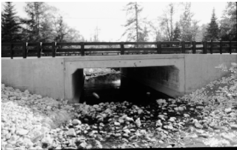
Figure 7. Low-profile box culvert.
