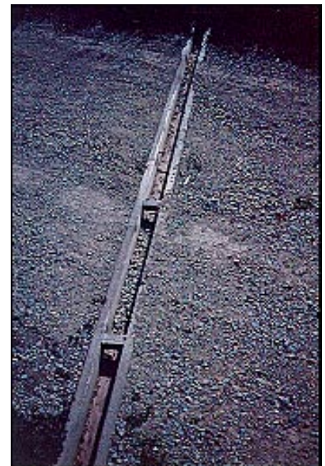
An open top culvert can be
