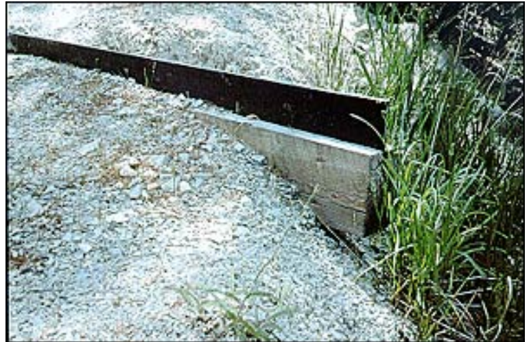
A deflector should be installed with approximately 3 inches of belting above the road surface.
